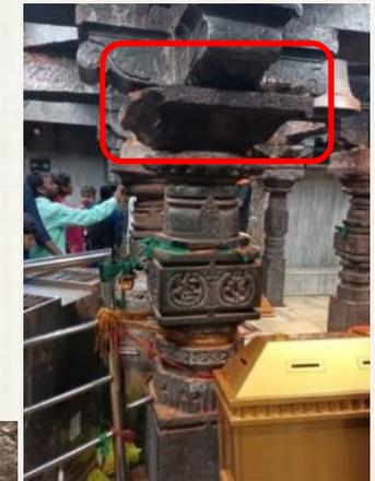
5. some parts of the column have got chipped off. Column capital edges are damaged at multiple locations.
