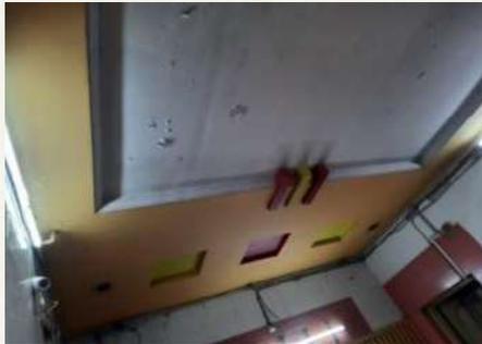
7. False ceiling installed . Walls clad with bright coloured ceramic tiles.
