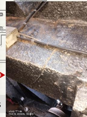
6. Cracks in beams
